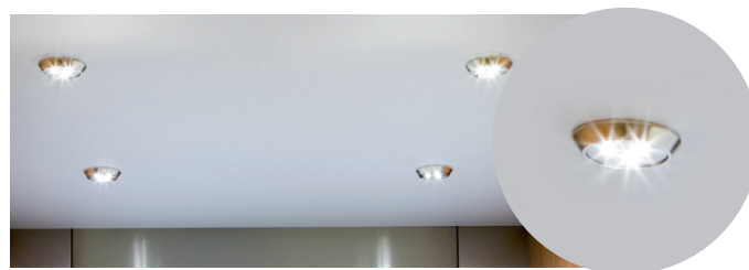
Ceiling with LED spots
